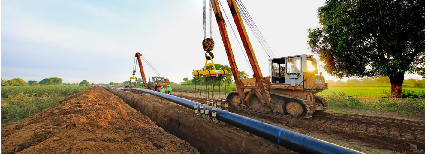
Pipeline laid for a cross - country project
