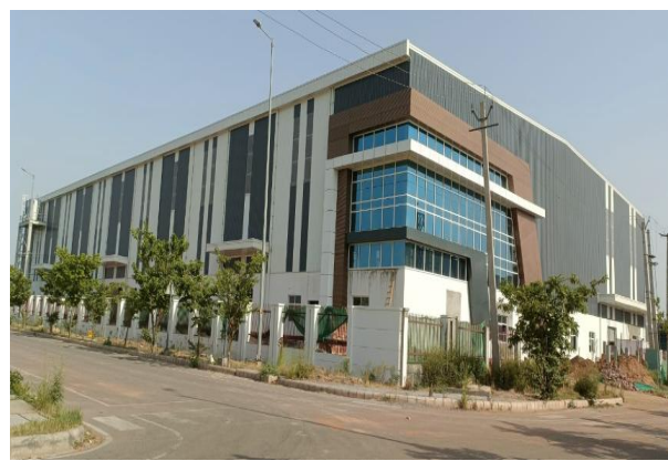
Total Weight of Building – 426.925 MT Jhajhhar, Haryana
