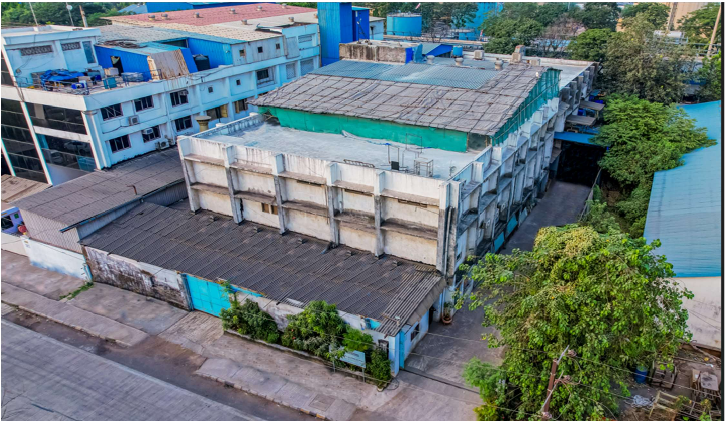
Registered Office and Manufacturing Unit-I (Outside)
