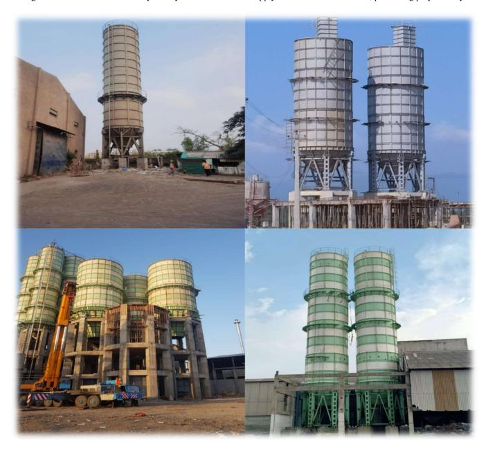
Artificial Sand Plant: An artificial sand plant, also known as a sand processing plant or sand washing plant, is a facility that processes sand for use in construction and other industries. Artificial Sand plants are designed to remove impurities such as dust, dirt, and organic matter from sand to produce high-quality sand for various applications.
