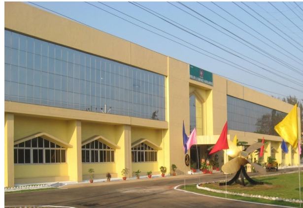
Steam System Repair Infrastructure at Naval Dockyard, Visakhapatnam
