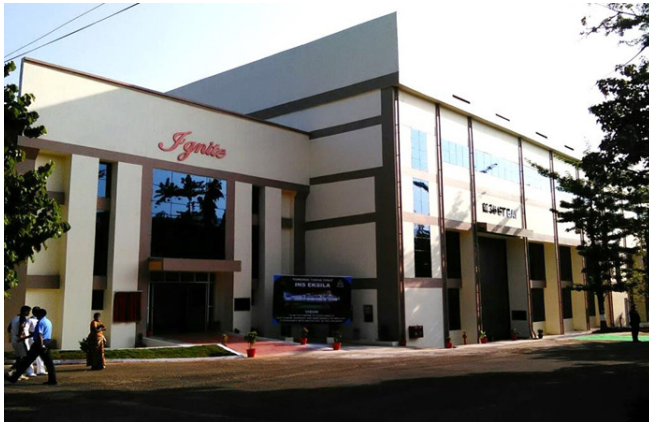
Overhauling facilities for M-36 GTs INS EKSILA, Visakhapatnam
