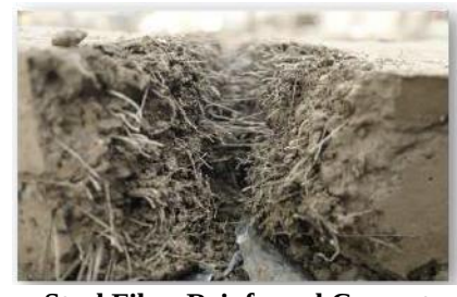
Steel Fiber Reinforced Concrete Flooring
