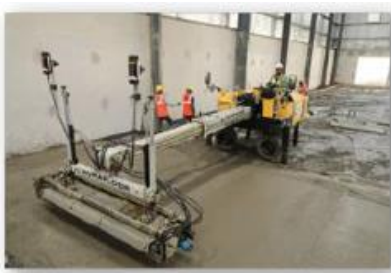
FM1/ FM2 Grade- Laser Screed Floors
